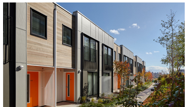
▲ T to B: Exterior, Suite Entry, Kitchen, Path
